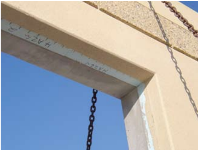
Flutes routed into the insulation layer of a precast concrete insulated sandwich wall panel can be seen in this panel example, which was used for a university dormitory project in Wisconsin.
